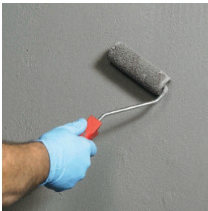
Apply first layer e.g. by roller or float covering the entire surface.
