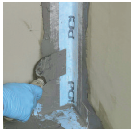
Install PCI Pecitape waterproofing tape in corners.
