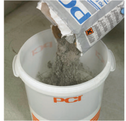
Add PCI Seccoral 2K Rapid powder.
