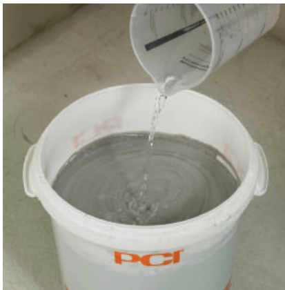
Add water for the application by roller (1 b).
