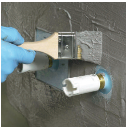
Fix PCI Pecitape 10 x 10 waterproofing collar and properly cover it with PCI Seccoral 2K Rapid.
